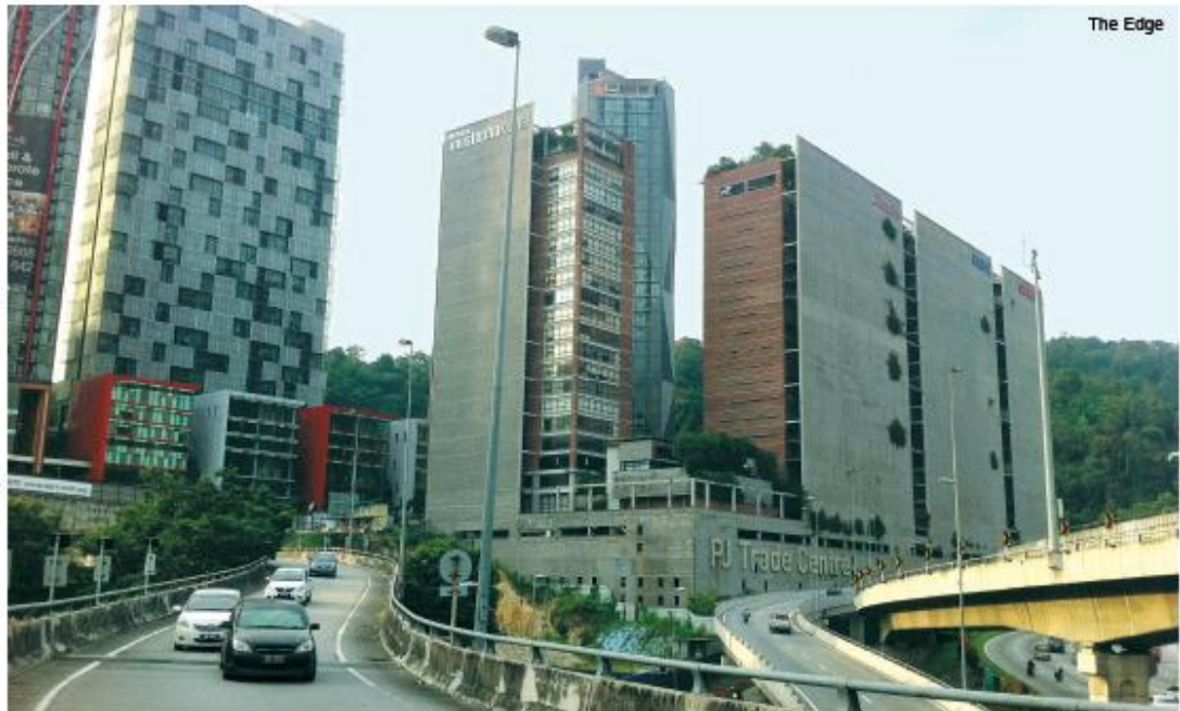
Menara Mustapha Kamal in Damansara Perdana
